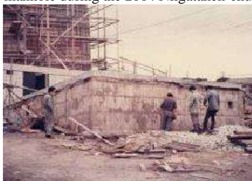
Fig5.4 Uplifted sewage tank during 1964 Niigata earthquake
