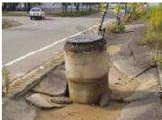
Fig5.3 Uplifted sewage manhole during the 2004 Niigataken-chuetsu earthquake
