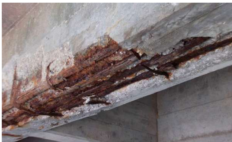
Fig5.11 Corrosion of RCC Structure
